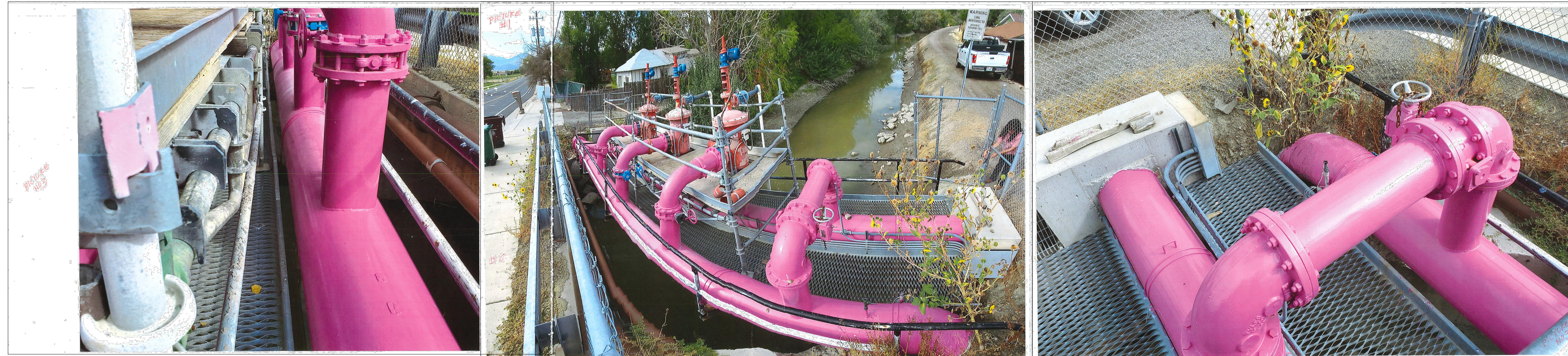
PICTURES OF EXISTING STRUCTURE
